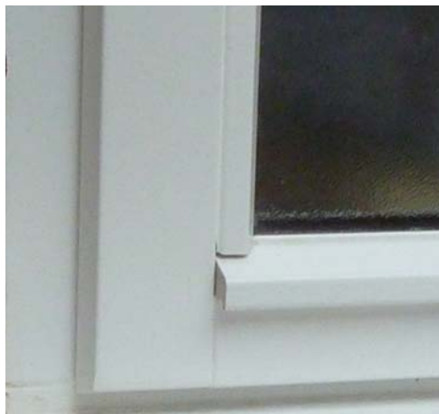
Modern storm-proof casement detail with incorrect rebated openers lipping over the face of the frame
